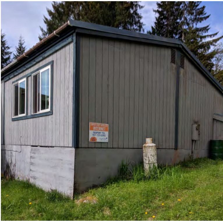
Figure 4: Side of building with Seaport internet sign
