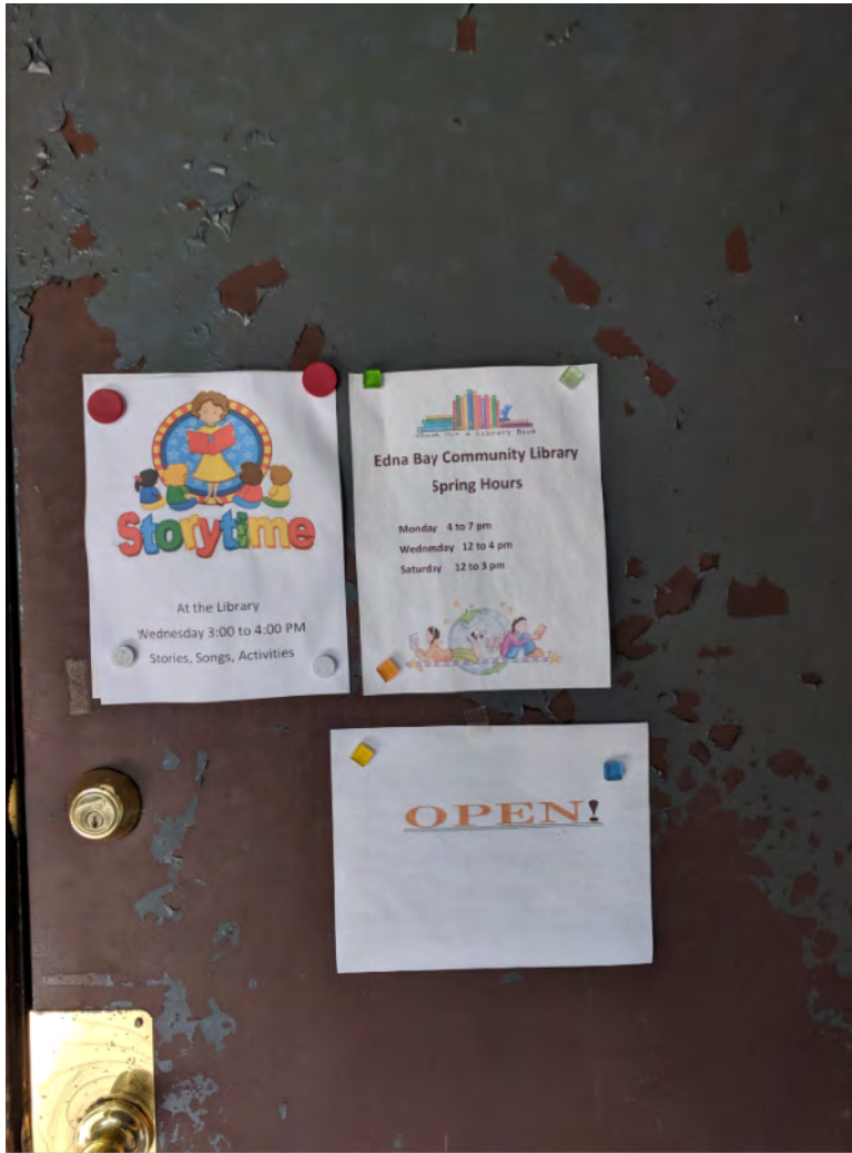
Figure 2: Actual door to library, inside front porch.
